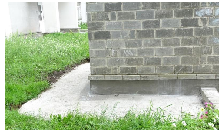
Reconstruction of concrete pavement of ventilation shafts
